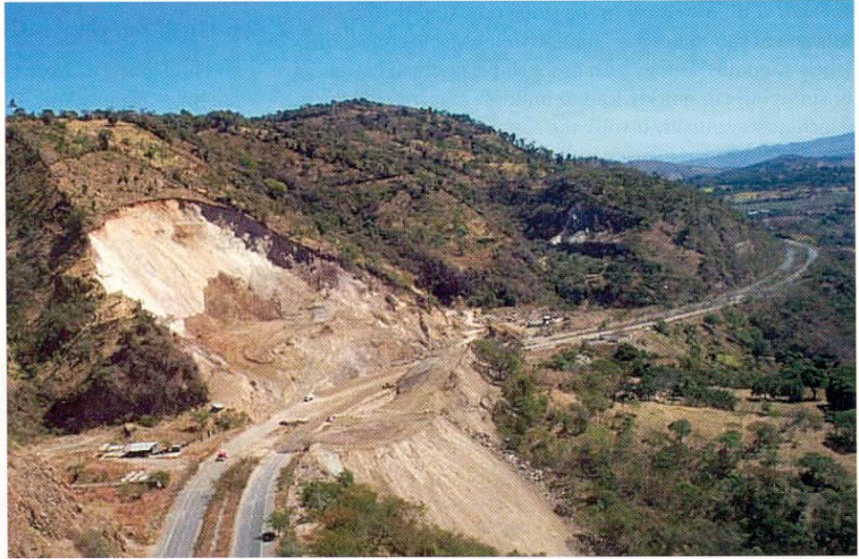
The San Vicente landslide (40km east of San Salvador on the Pan American Highway) was triggered by the January 2001 El Salvador Earthquake and covered the highway with 20 meters of debris.
